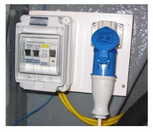
Protection is easily achieved using a conventional domestic consumer unit. The ideal unit for this purpose is one of the small consumer units specifically designed for outbuildings and garages. These normally come ready fitted with a 30mA RCD, one 6amp MCB (intended for the lighting circuit in the outbuilding), and one 16 amp circuit breaker (intended for the ring main in the outbuilding).
